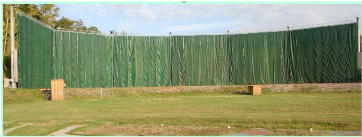
Figure 1-5: Example for a vertical barrier in a clay shooting range (Herrmann, 2013)
