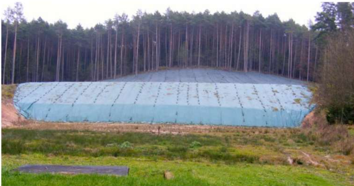
Figure 1-7: Example of a horizontal barrier (Bavarian LFU, 2014a)
