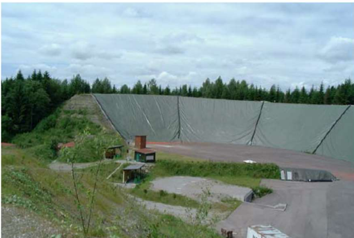
Figure 1-8: Example of a range with both a horizontal and vertical barrier (Bavarian StMLU, 2003)
