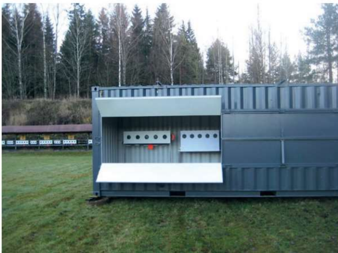
Figure 1-12: Example of a prototype of biathlon target equipment and trap chambers installed in a shipping container (Kajander and Parri, 2014)
