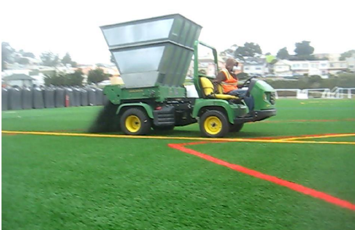
Figure A 9: Semi-mechanised application of infill
