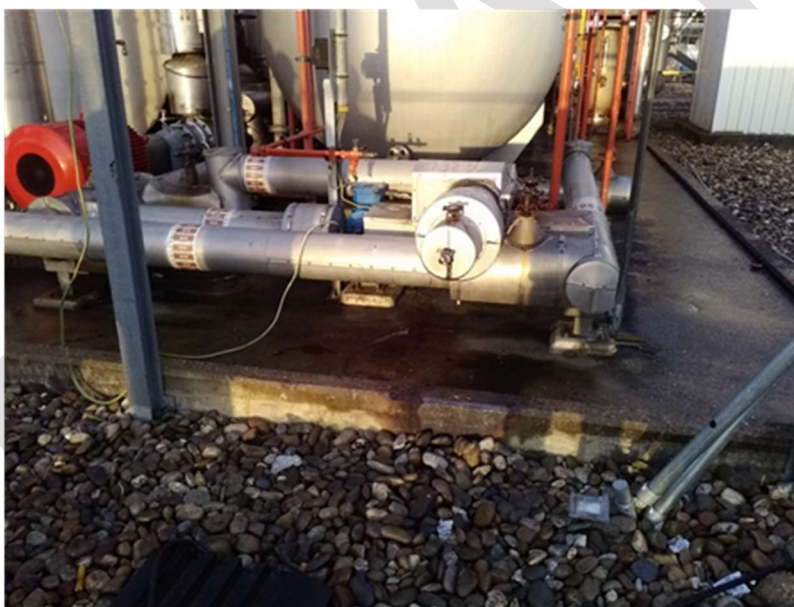
Figure 4. Soil sample point in Site S-01
