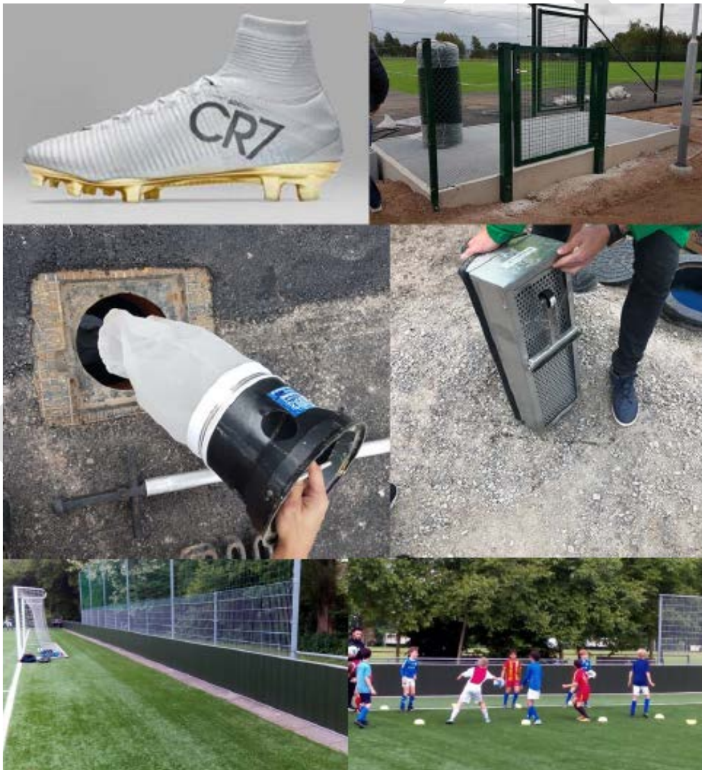
Figure 19: Footwear with integrated socks, entrance with player-cleaning-area, special drains with filters/interceptors. Source: BIR Tyre & Rubber Com (2019).
