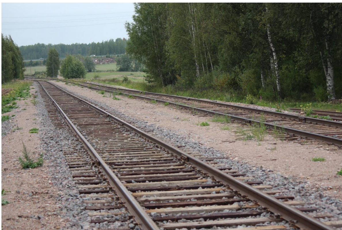
Figure B - 6: Reused wooden sleepers, Lapinjärvi, Finland, August 2021 (source: FTI Finland)
